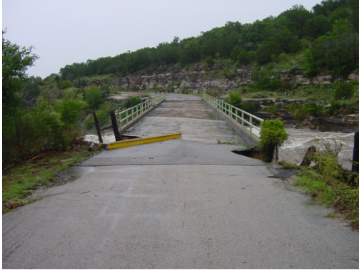
Starcke Dam access road, damaged by flooding on Flat Rock Creek
