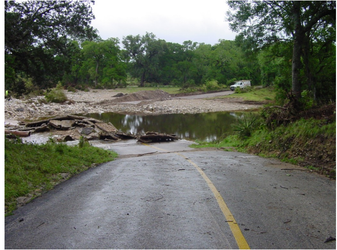
Washout of FM 2147 at Double Horn Creek southeast of Marble Falls
